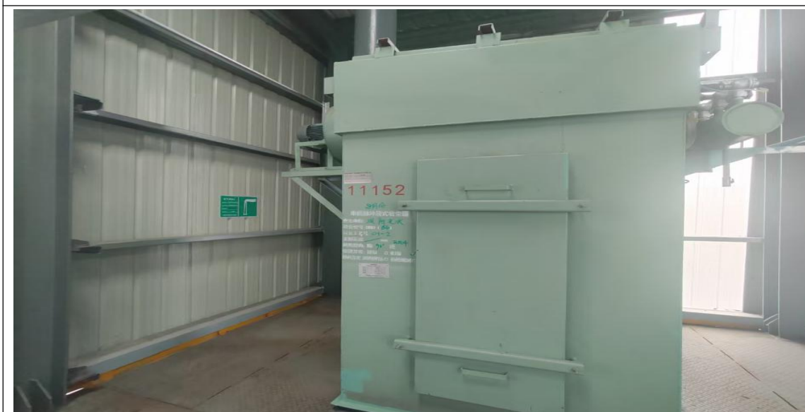
1#纯碱库顶废气袋式除尘+34.5m 排气筒 (DA010)
